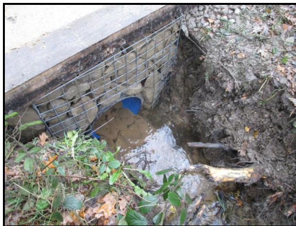
New culverts and drainage at Baron Fields – December 2019
